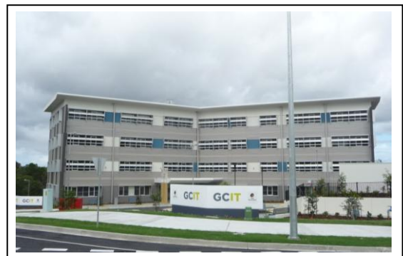
The recently opened Coomera TAFE will offer vocational training in information technology, the creative industries and computer-based training for construction/engineering courses
